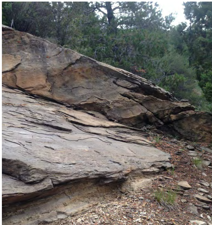
Photo 3. Stress relief exfoliation in high bitumen sandstone units.
